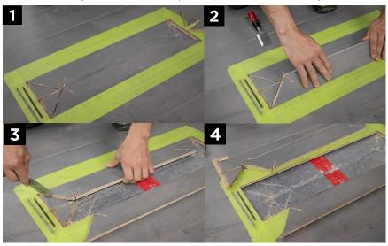
Vacuum the opening. If the membrane is damaged add some tape to fix, if needed.
