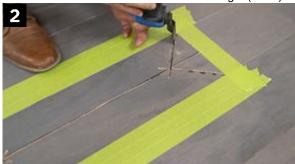
• Next, make one long cut near the groove side, about 1/8 (3-4 mm) from side (d).
